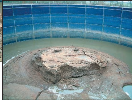
Below: Solids in the pig slurry store in December 2008
